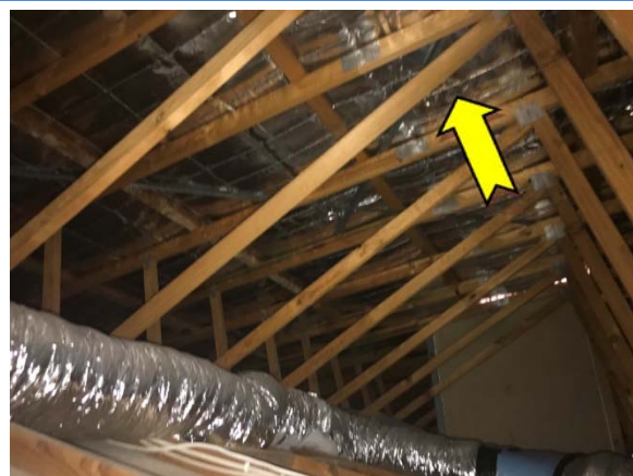
Photo 12. Interior, throughout, roof space – suspected SMF sarking insulation.
