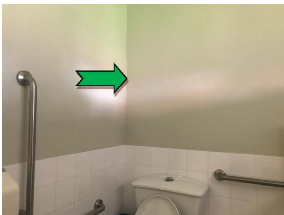
Photo 5. Interior, staff WC, throughout walls – non asbestos-containing fibre cement sheeting.
