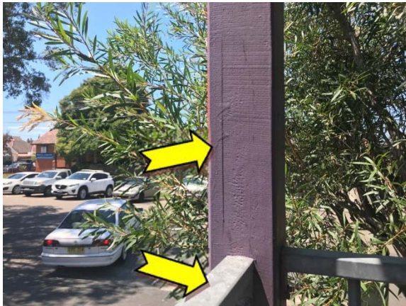
Photo 15. Exterior, throughout, verandah, timber beams - suspected lead-containing purple (light & dark) upper paint systems.
