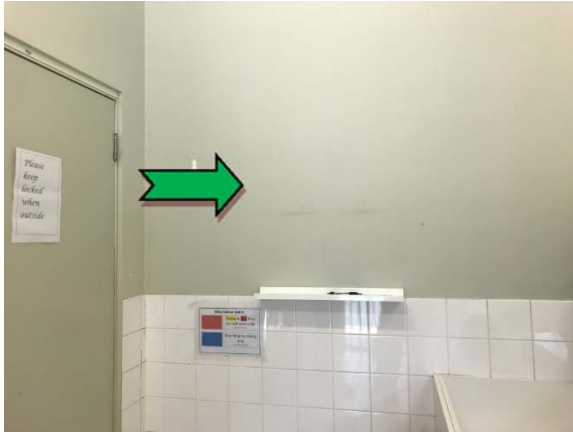
Photo 7. Interior, toilets 2, throughout, walls – non asbestos-containing fibre cement sheeting.
