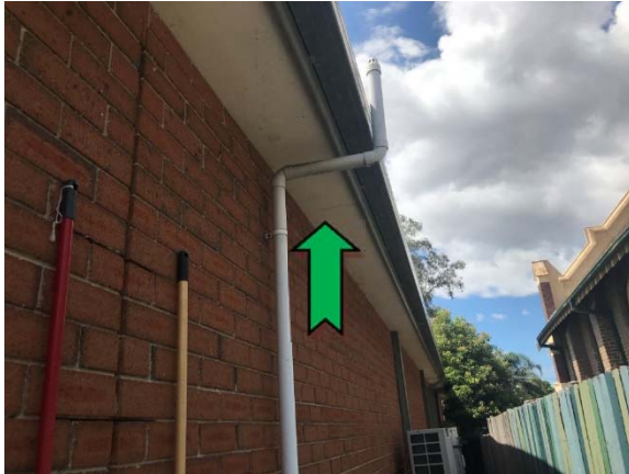
Photo 1. Exterior, south elevation, throughout, eaves – non asbestos-containing fibre cement sheeting.
