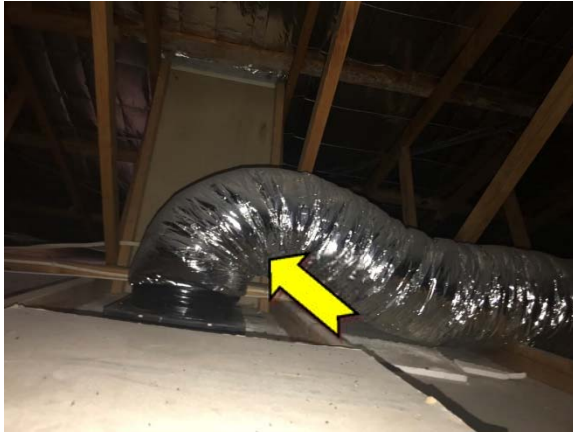
Photo 13. Interior, roof space, flexible ductwork – Suspected SMF internal insulation.
