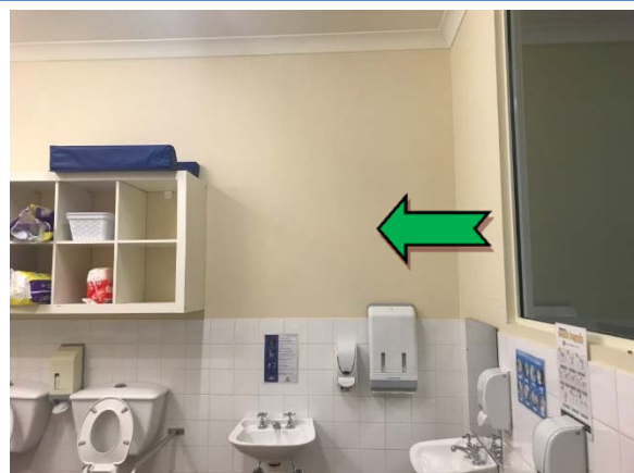
Photo 6. Interior, toilets 1, throughout walls – non asbestos-containing fibre cement sheeting.
