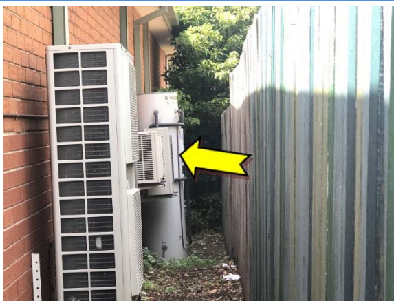
Photo 11. Exterior, south elevation, hot water heater – suspected SMF internal insulation.
