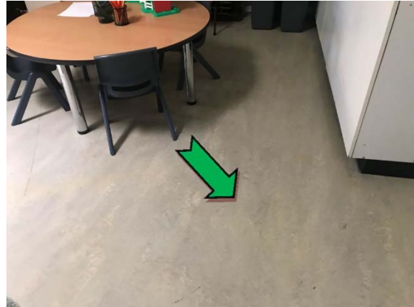
Photo 8. Interior, playroom 1, throughout, floor coverings – suspected non asbestos-containing vinyl sheeting.
