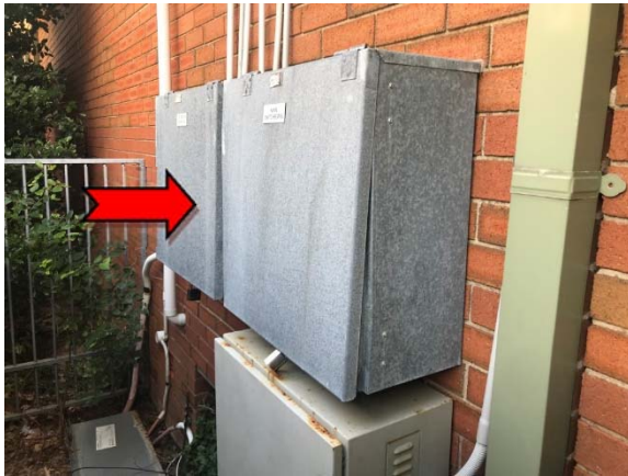
Photo 3. Exterior, south elevation, electrical backing board – suspected asbestos-containing bituminous backing board.
