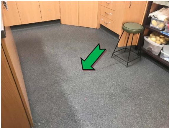
Photo 9. Interior, kitchen, throughout, floor coverings – suspected non asbestos-containing vinyl sheeting.
