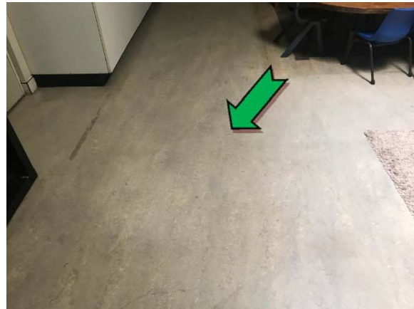
Photo 10. Interior, playroom 3, throughout, floor coverings – non asbestos-containing vinyl sheeting.
